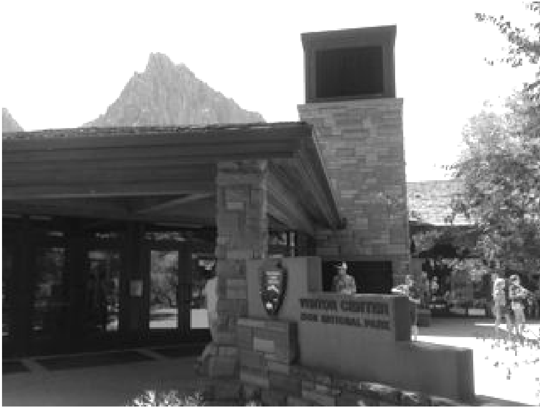
Figure 4. Wind catcher tower at Zion National Park Visitors Center.
