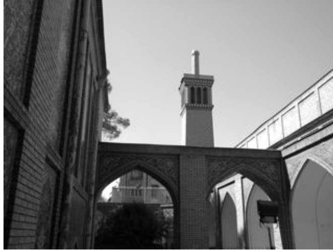
Figure 1. BAD GIR tower in Tehran, Iran.
